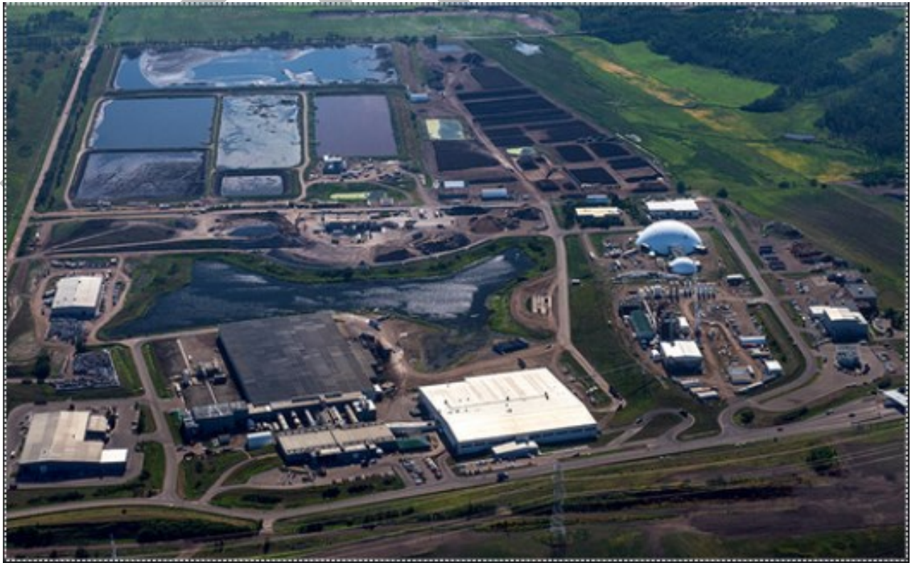
Figure 6-5 Edmonton Resource Recovery Facility
