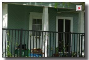
Siding applied in an incompatible herringbone pattern
