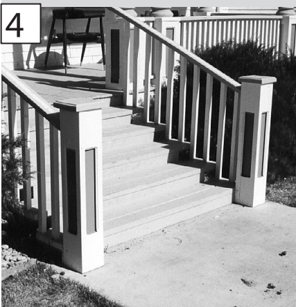
After: Handrail repaired and the post replaced in kind
