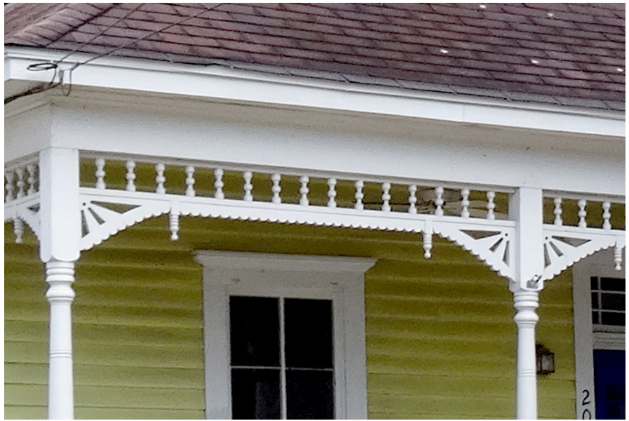
Key, character-defining features include the porch columns, spindles and jigsaw trim, double-hung window and casing, and wood cladding.
