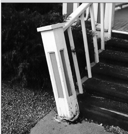
Before: A deteriorated handrail
