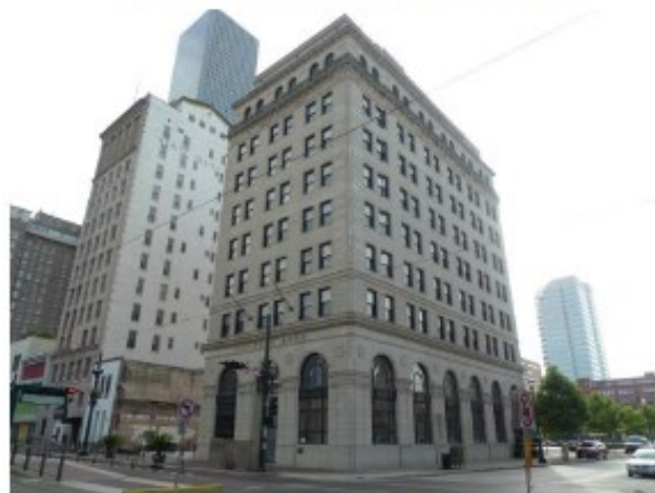
Contributing structures along the 400 Block of Main
