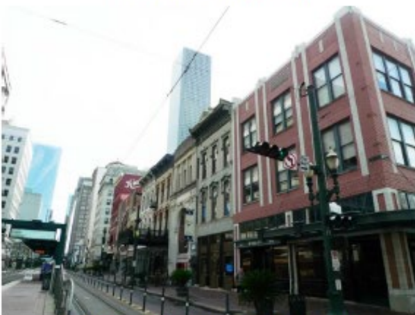
Contributing structures along the 300 Block of Main
