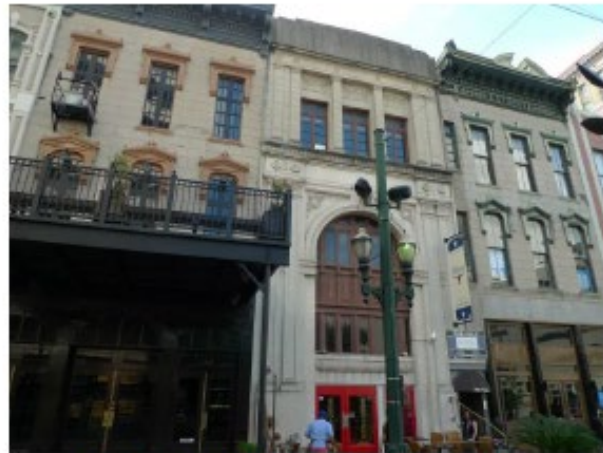
Contributing structures along the 300 Block of Main
