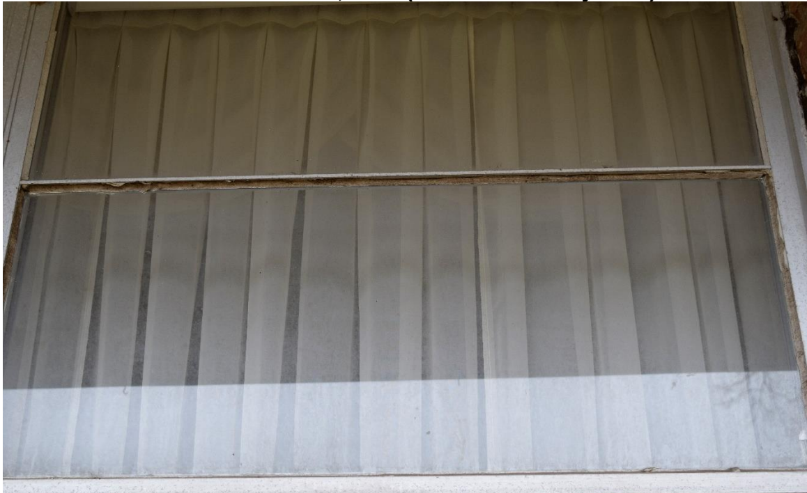
Windows to the Right-Hand Side of Structure
