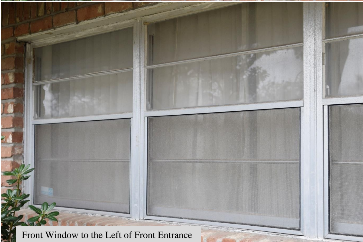
Front Window to the Left of Front Entrance
