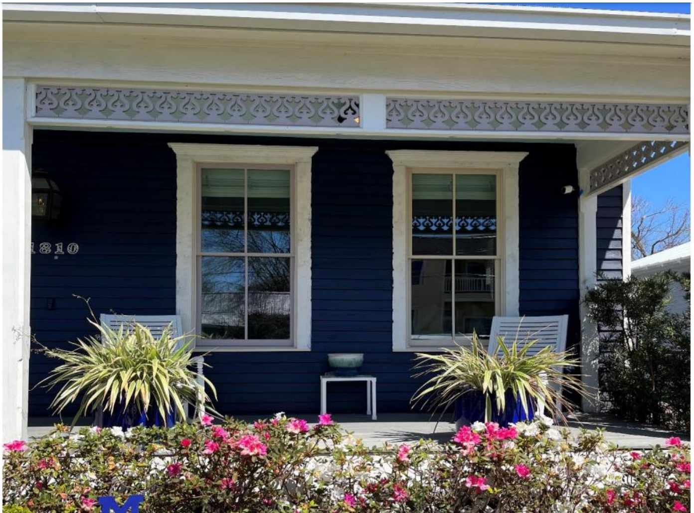
Figure 5 - Applicant Supplied Photo with New Windows on Porch
