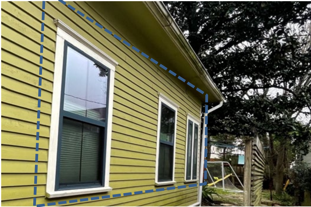
Non-original, REPLACEMENT windows
