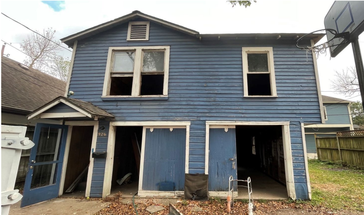
GARAGE – FACING COURTLANDT STREET
