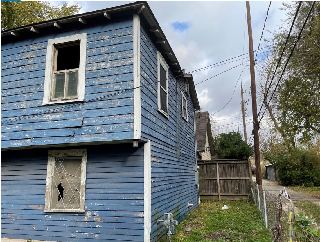
HARRIS COUNTY ARCHIVE BLA – C.1950 – HOUSE RAISED TO ACCOMMODATE GARAGE
