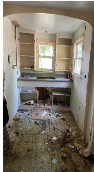
Existing First Floor Kitchen at Garage Structure
