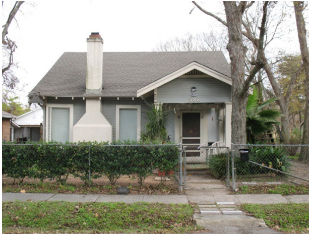
532 Granberry– Contributing – 1925 (next street)
