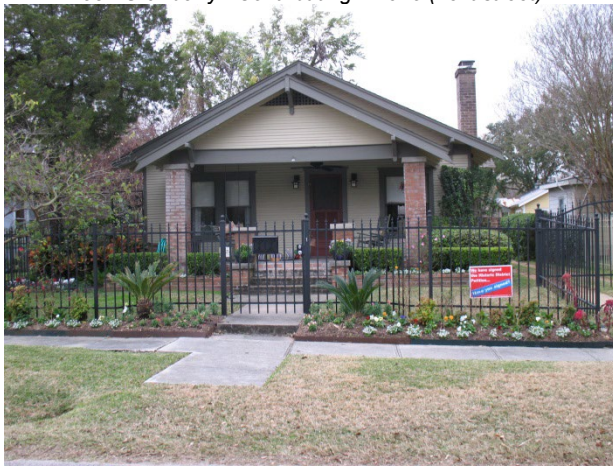
527 Granberry– Contributing – 1923 (next street)
