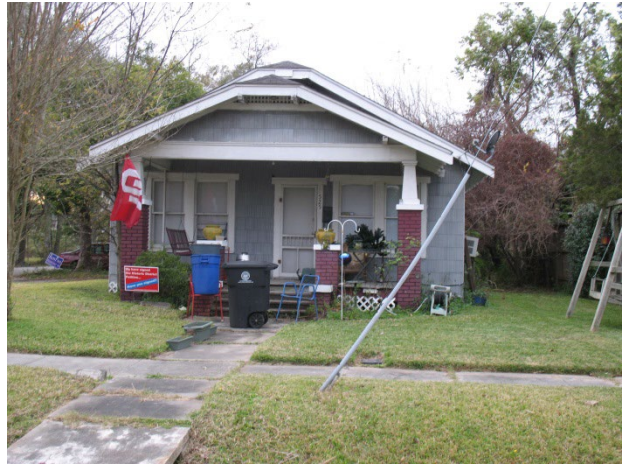
525 Granberry– Contributing – 1923 (next street)
