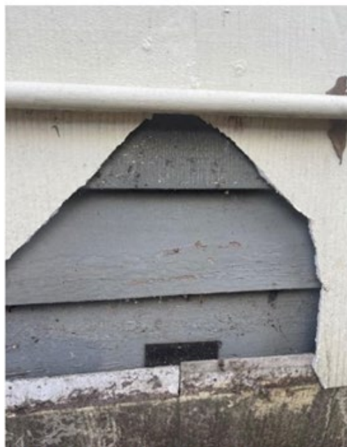
Original Siding underneath the existing siding.
