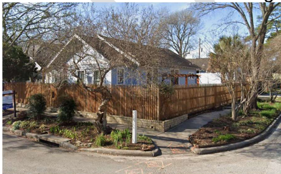
1545 Alston Street - Contributing
