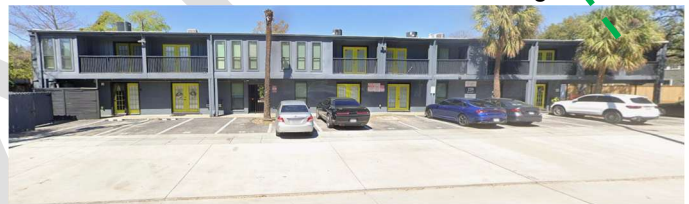
239 Emerson St – Non-contributing
