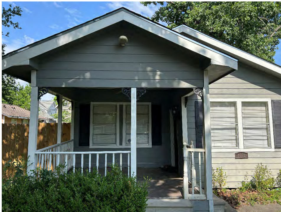
Figure 2 - Non-Contributing House at Site to be Razed
