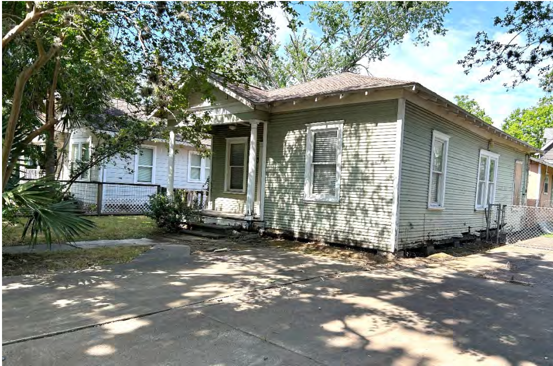
Figure 3 - House to the Left of Site
