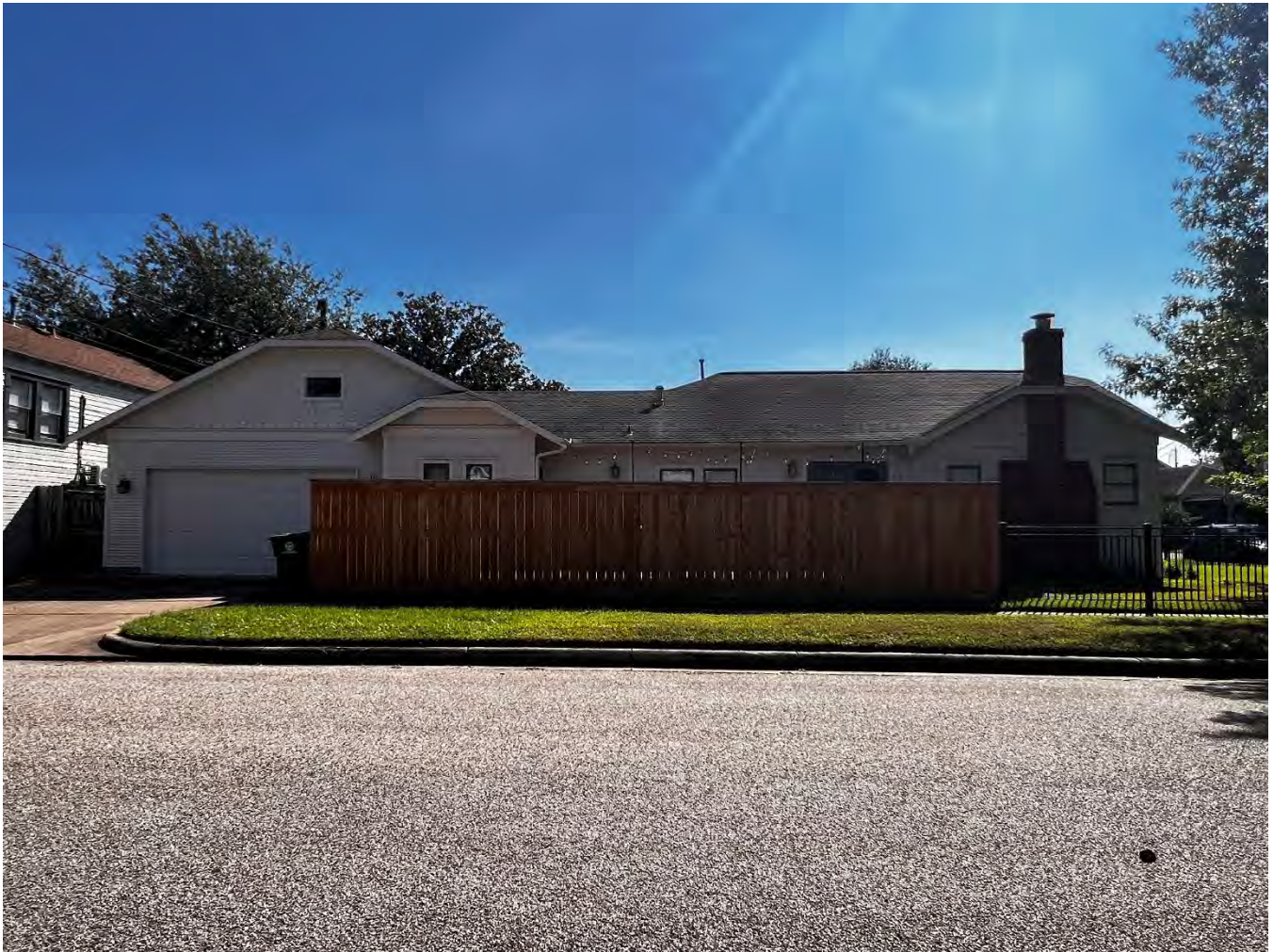
Figure 2 - Current Image Left/West Elevation
