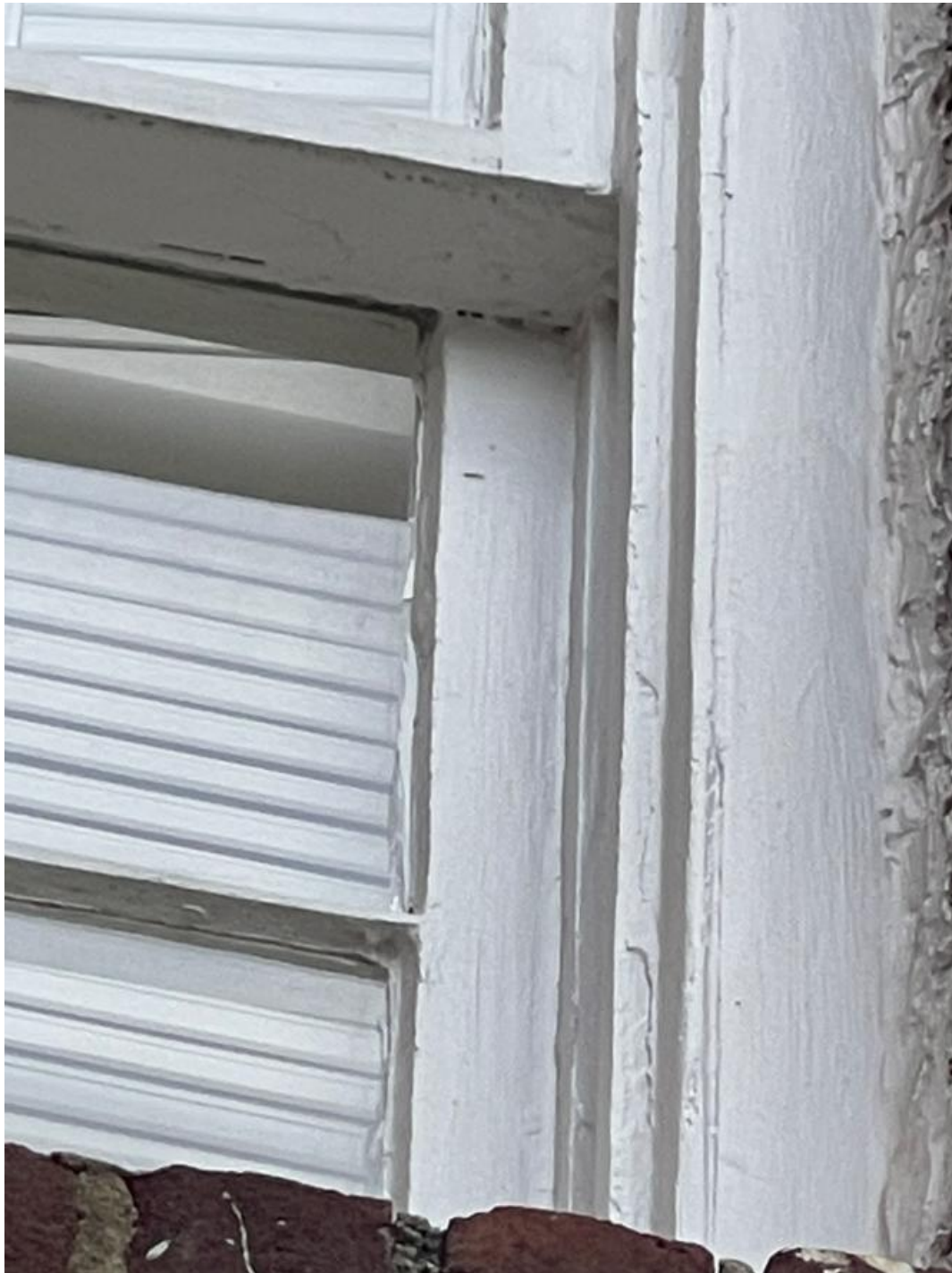
Repeated water damage, to window and brick, main house East Elevation, 2 nd story front.
