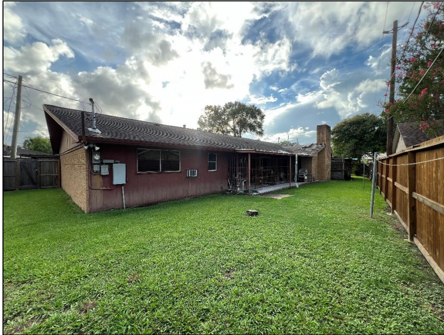
Photograph 3: View of rear elevation of the residence.
