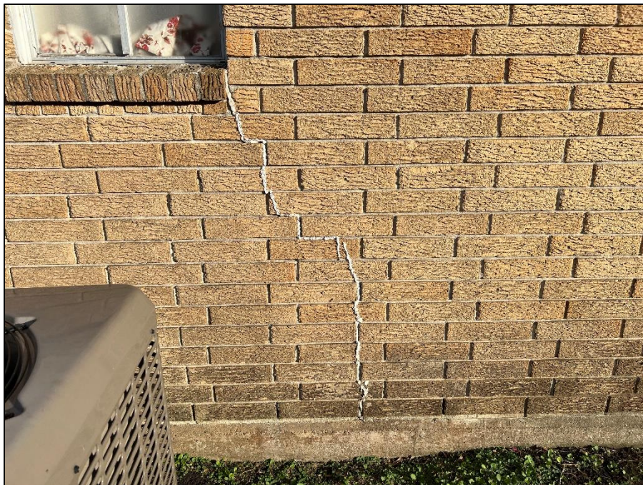
Photograph 12: Typical view of historical mortar repair.
