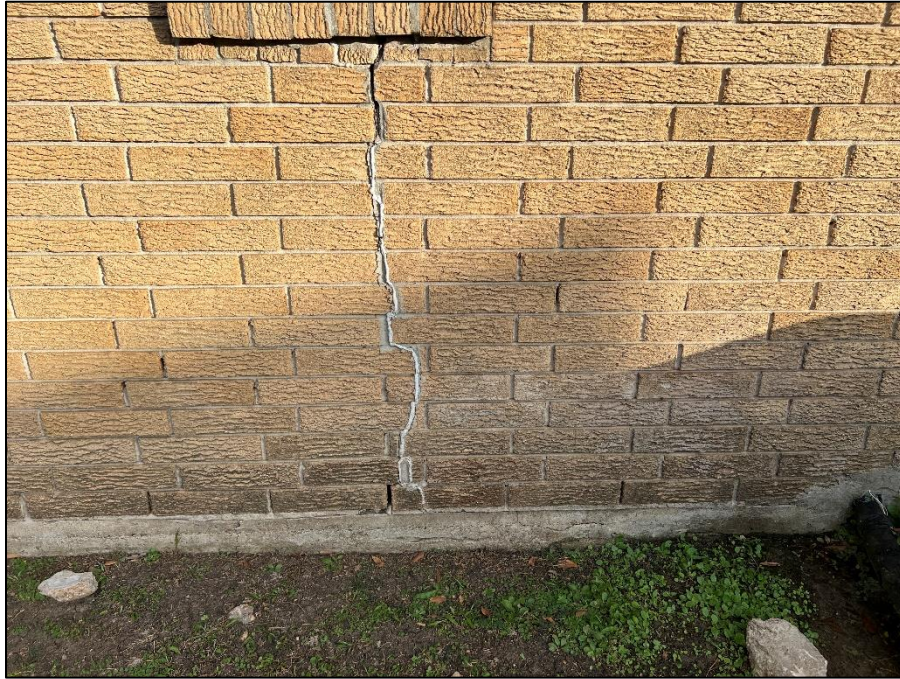
Photograph 13: Typical view of historical mortar repair.
