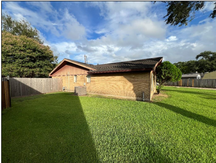
Photograph 4: View of left elevation of the residence.
