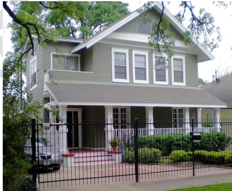
705 Marshall Street – Non-Contributing -- 1917
