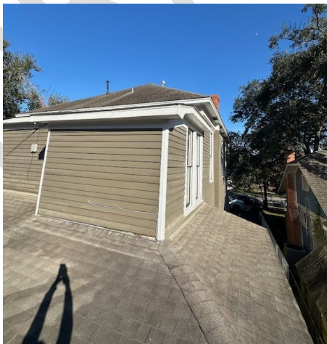
SOUTHWEST (REAR/LEFT) CORNER BUMPOUT
