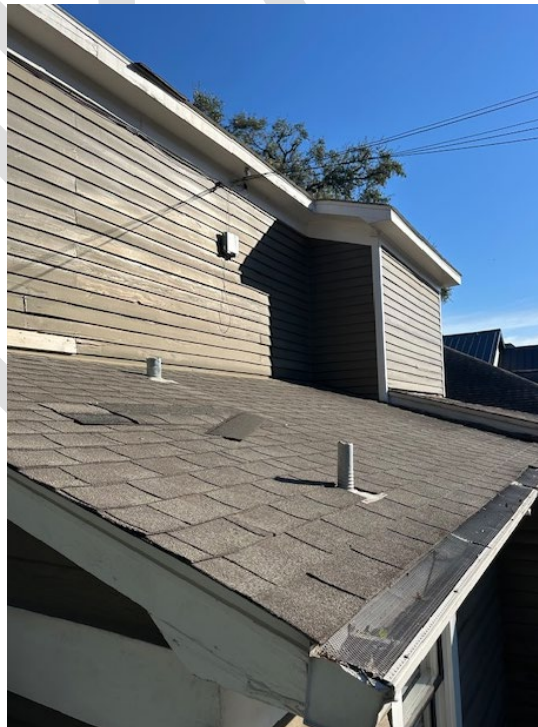
OBLIQUE VIEW OF REAR BUMPOUT AND ROOFLINE
