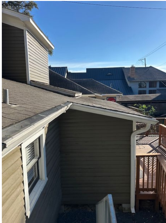
OBLIQUE VIEW OF REAR BUMPOUT AND ROOFLINE
