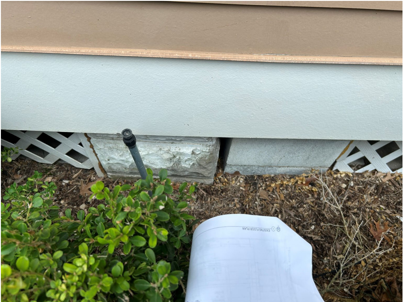
Figure 7 - Seam area Original House to Addition
