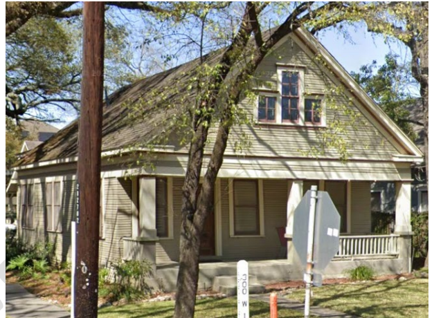
321 W 13 th St – Contributing – 1915 Located two doors down to left of structure
