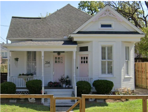
314 W 13 th St – Contributing – 1905 Located across the street from structure
