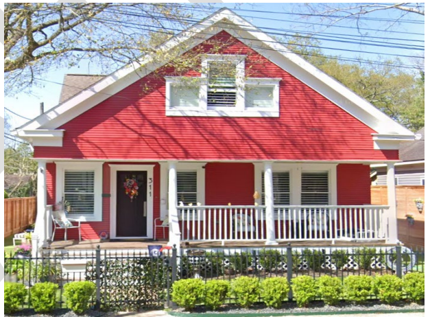
311 W 13 th St – Contributing – 1915 Located to the right of structure
