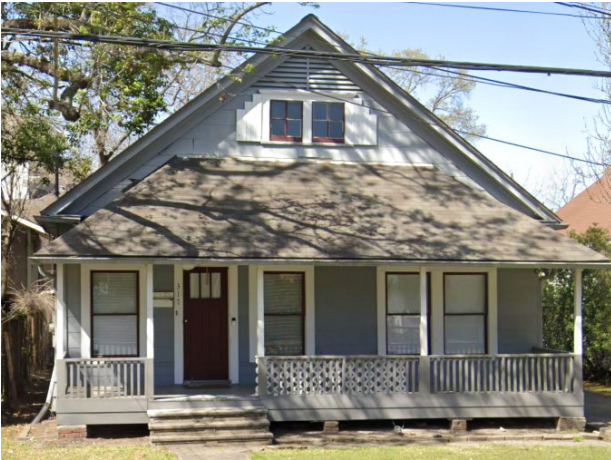
317 W 13 th St – Contributing – 1915 Located to the left of structure
