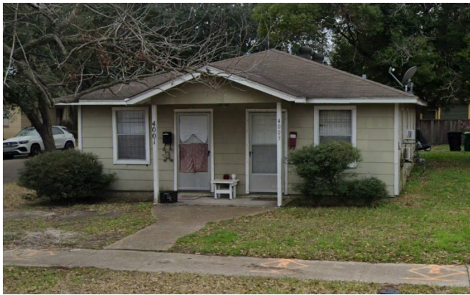
Figure 3- 4001 Michaux - next door neighbor
