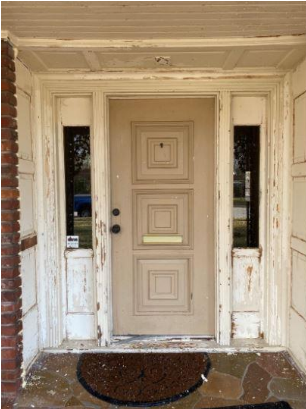
Door Before Replacement
