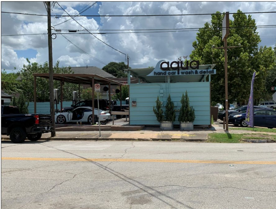
EXISTING CAR WASH BUILDING
