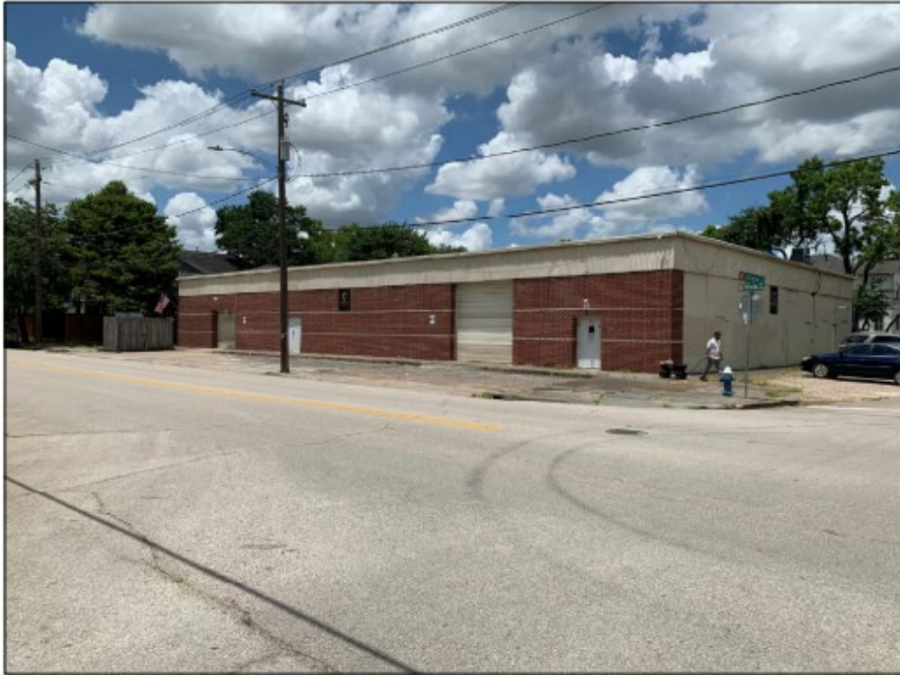
EXISTING 3400 WHITE OAK, CONTRIBUTING, ESTIMATED HEIGHT 18'-0", MIXED BRICK, CONTINUOUS EXTENDED PARAPET CAP
