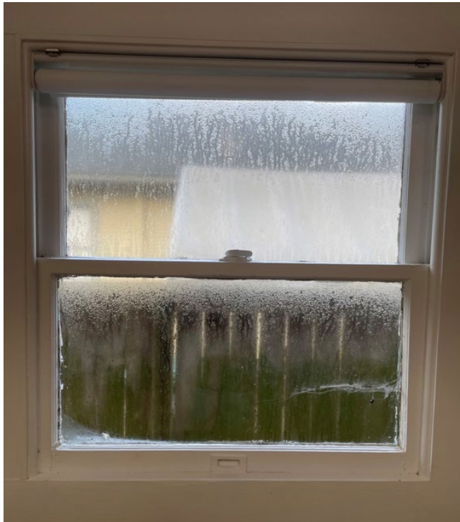
WINDOW 13 (WEST AT REAR) – TO BE REMOVED & COVERED WITH SIDING
