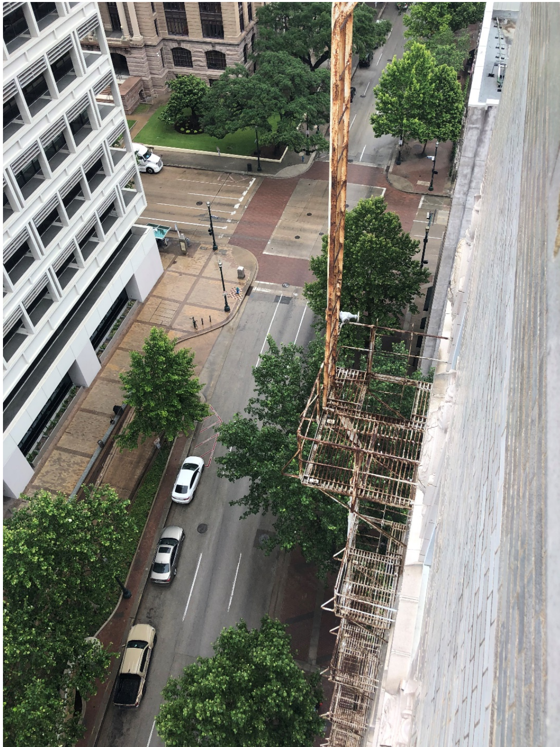
Photo 4: Another view of the fire escape.
