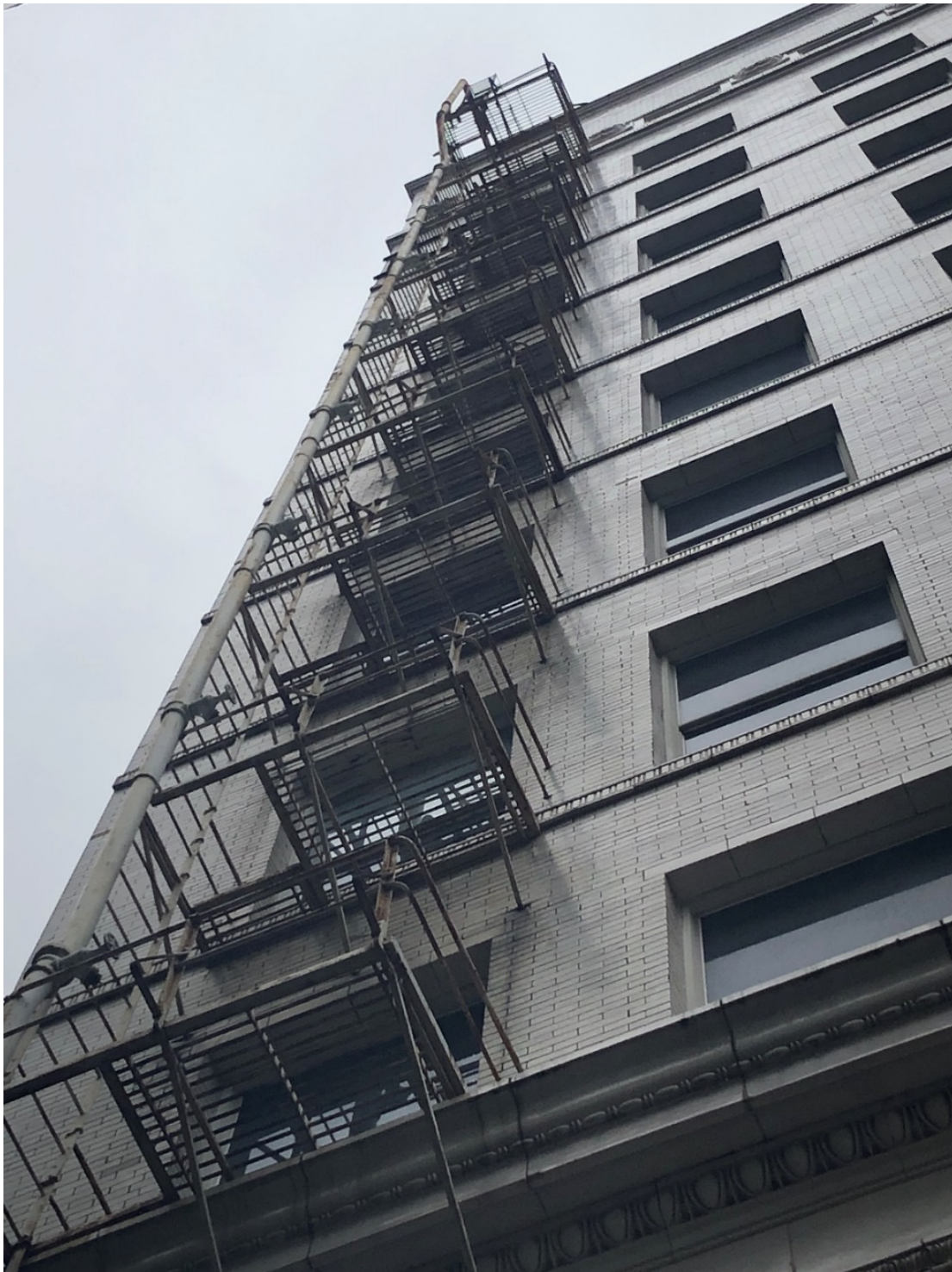
Photo 2: Closer view of fire escape to be removed.
