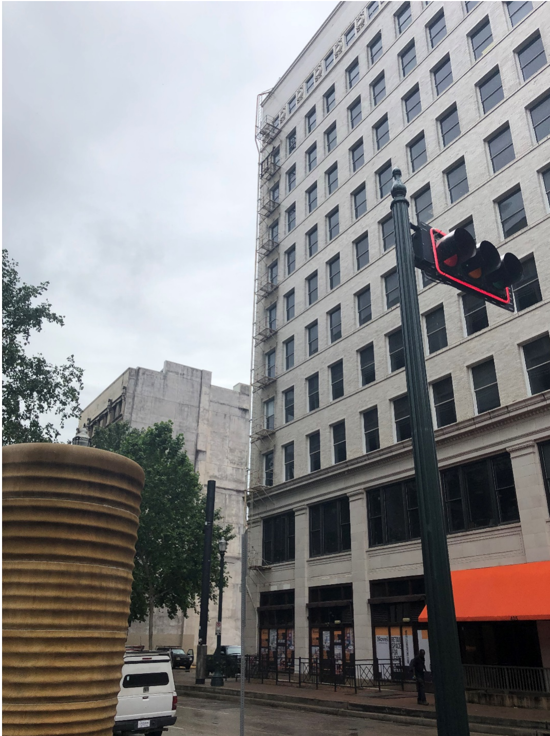
Photo 1: Far view of fire escape.
