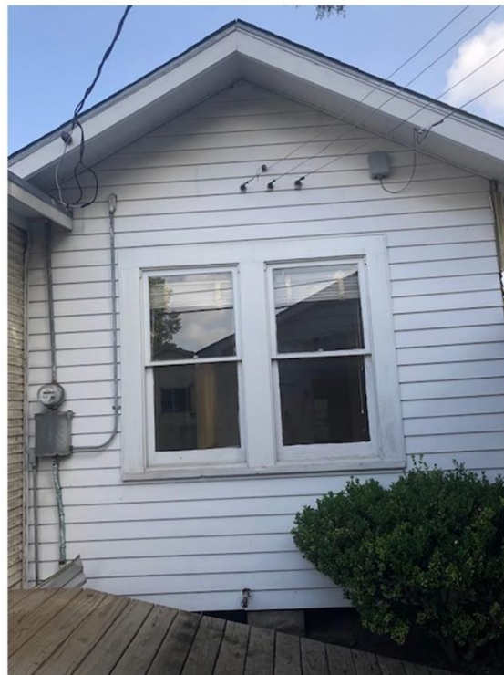
Back (south side) of house, original portion
