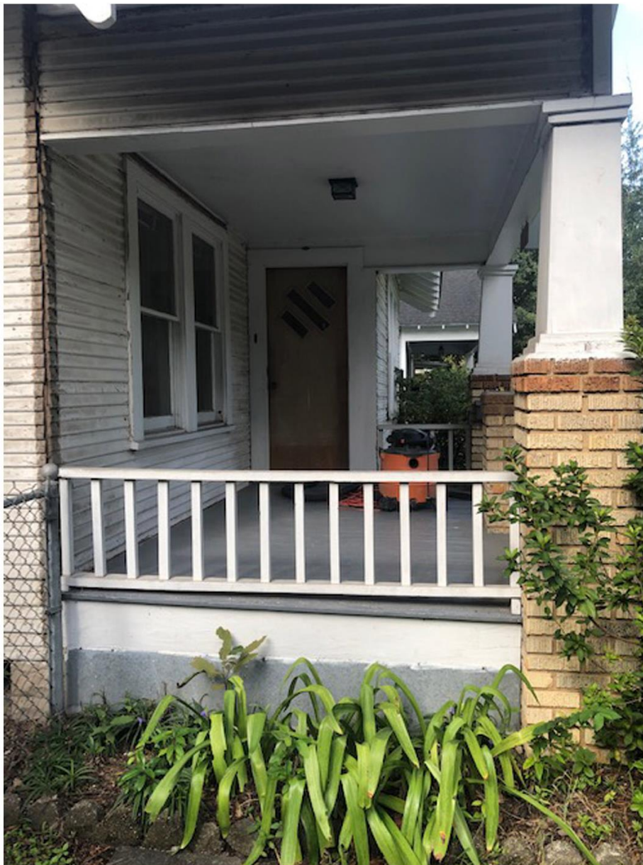
Front porch where plywood will be removed to expose original beadboard
