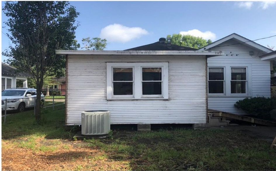
Back (south side) of house, existing addition
