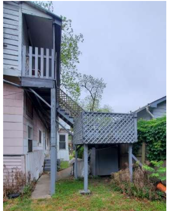
Rear View (non-original addition)
