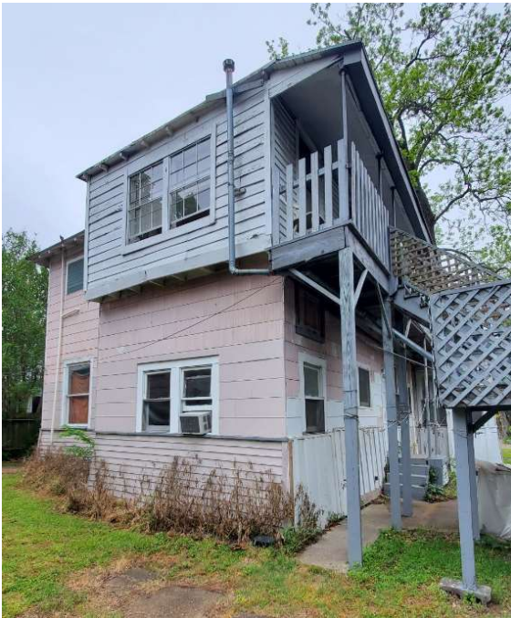
Rear View (non-original addition)
