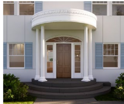
RENDERING OF PROPOSED DESIGN - PANELED WOOD DOOR WITH NEW SIDELIGHTS & TRANSOM TO MATCH HISTORIC DETAILS & PROPORTIONS
