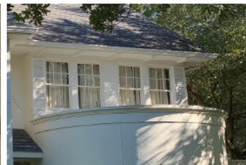
EXISTING CONDITIONS TODAY - 1980s ADDITION WINDOWS
