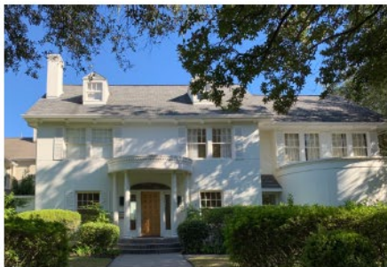
EXISTING SHINGLE ROOFING ON HISTORIC PORTION
