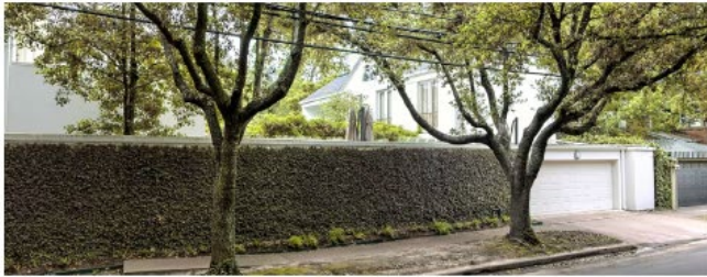
EXISTING CONDITIONS TODAY - DETACHED GUEST QUARTERS VIEWED FROM DUNLAVY NOTE: EXPOSED SOUTH-FACING JULIETTE BALCONIES
