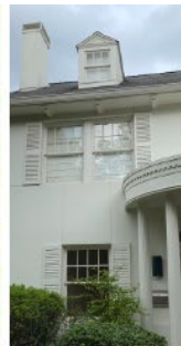
EXISTING CONDITIONS TODAY, WHITE STUCCO & SHUTTERS
