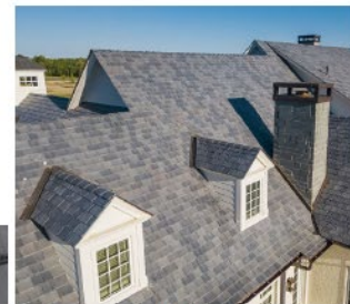
PROPOSED SYNTHETIC SLATE MATERIAL TO REPLACE EXISTING COMPOSITION SHINGLE ROOFING ON HISTORIC PORTION, REAR BALCONY ROOF, & DETACHED GUEST QUARTERS
