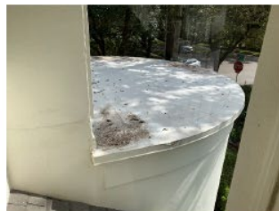
EXISTING CONDITIONS TODAY - MEMBRANE ROOFING
