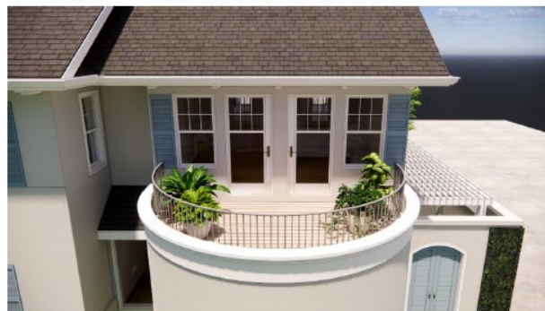
RENDERING OF PROPOSED DESIGN - RAILING INSET FROM EDGE. CENTER WINDOWS REPLACED WITH NEW WOOD DOORS TO MATCH EXISTING WINDOW PROPORTION & DETAILS.
