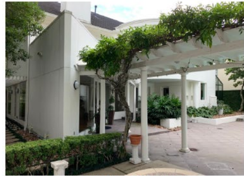
EXISTING CONDITIONS TODAY - TRIANGULAR ROOM WITH BALCONY ABOVE
