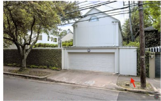
EXISTING CONDITIONS - GARAGE WALL
