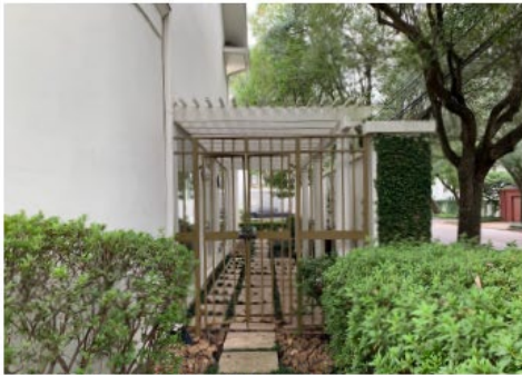
EXISTING CONDITIONS - PERIMETER WALL & METAL GATE
