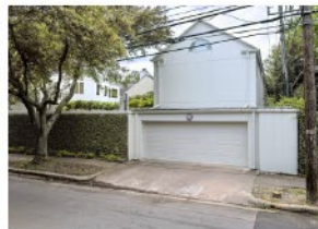
EXISTING CONDITIONS, VIEWED FROM DUNLAW ST
