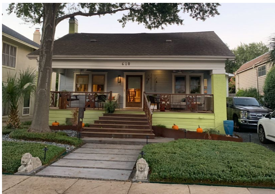
EXISTING (WORK ALREADY COMPLETED) 2019
