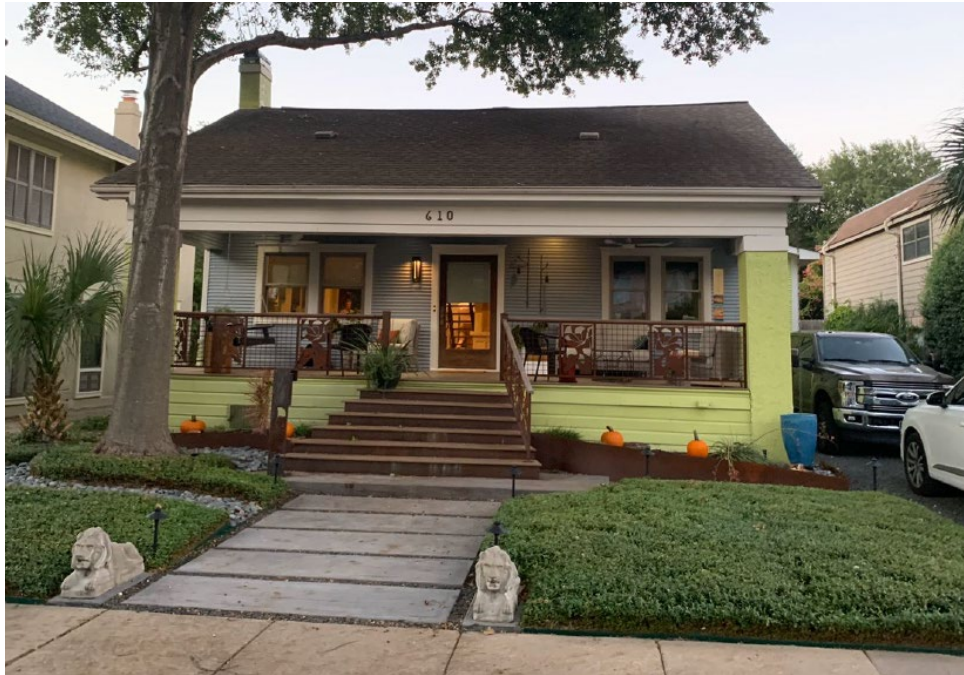
EXISTING (WORK ALREADY COMPLETED) 2019
