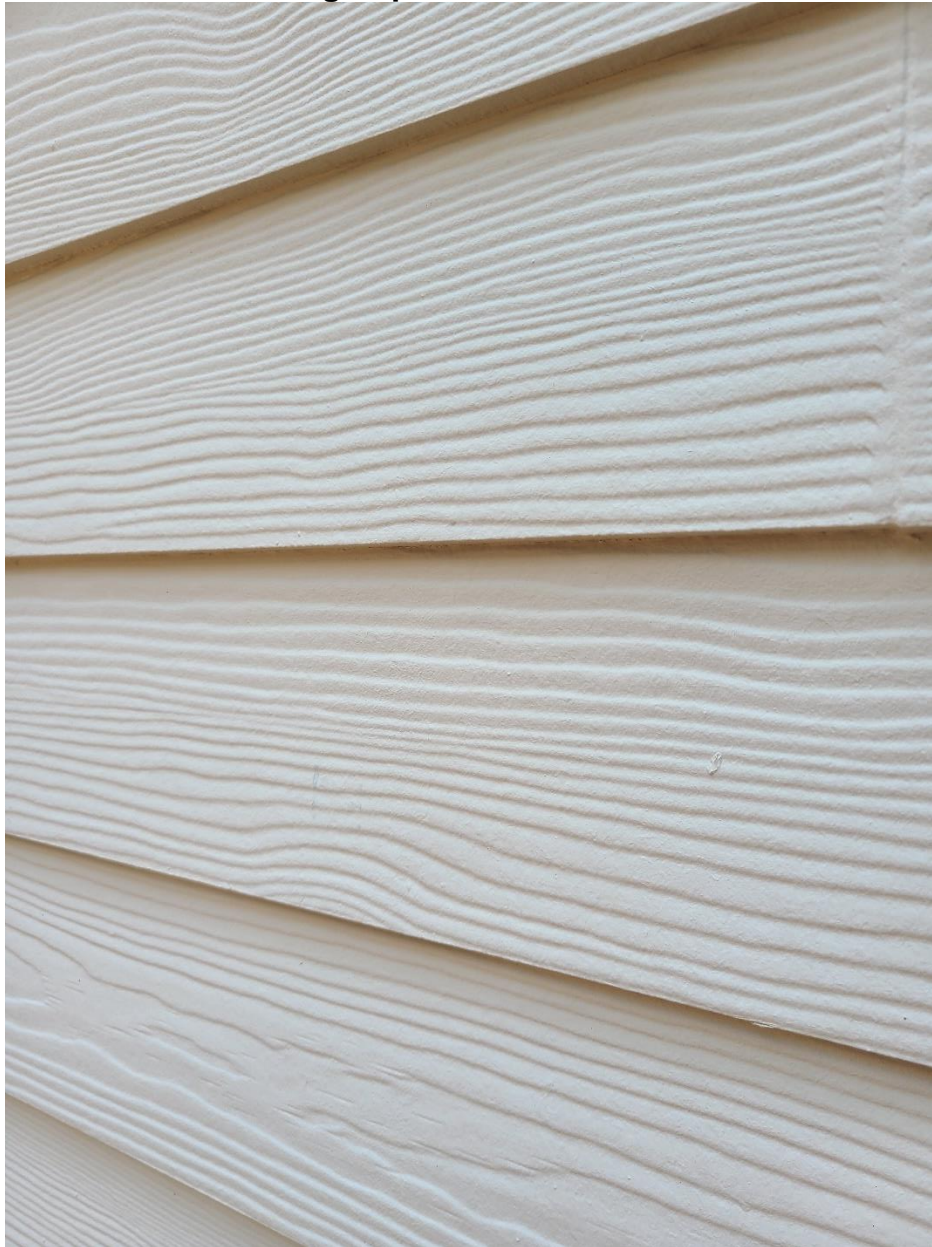
Close up of textured cementitious siding used for repair
