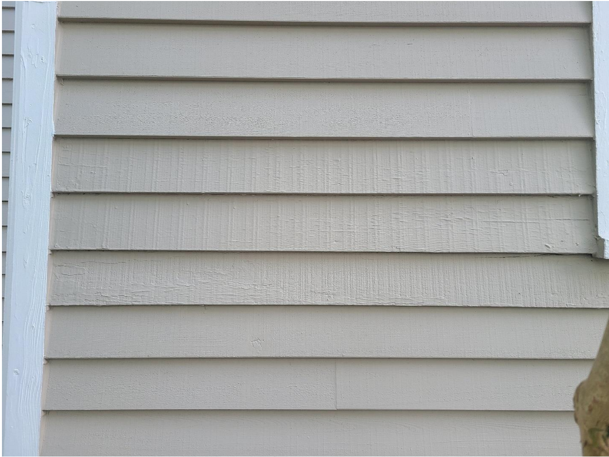
Close up of different materials used to replaced siding
