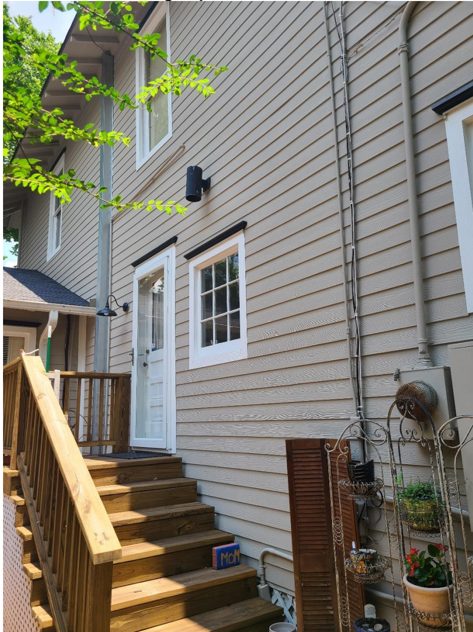
Siding Replaced on West Side
