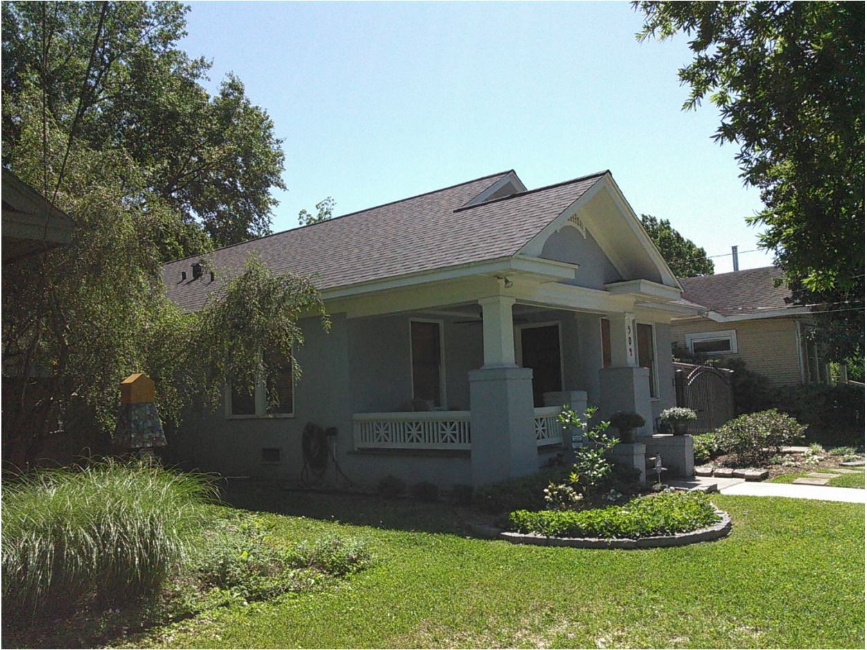
East side-front view.
