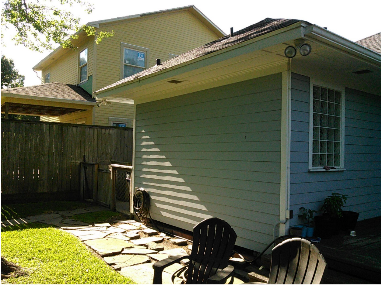
South side facing back yard – previous addition, partial view.
