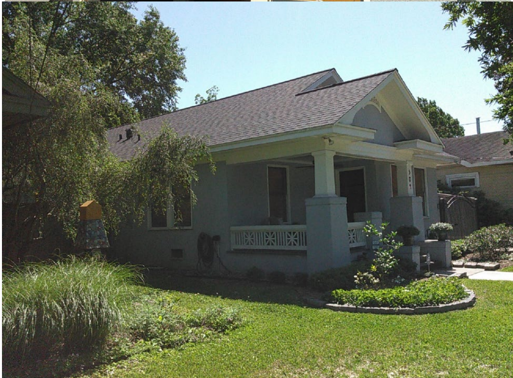
East side-front view.
