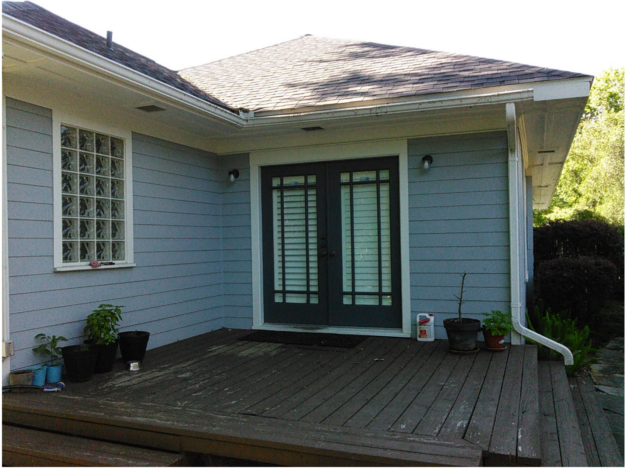
South side facing back yard – previous addition/deck, partial view.
