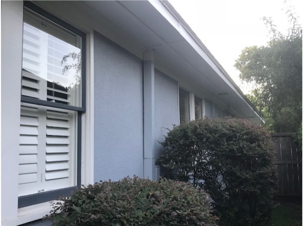
East side showing fascia/stucco transition between original and previous addition.
