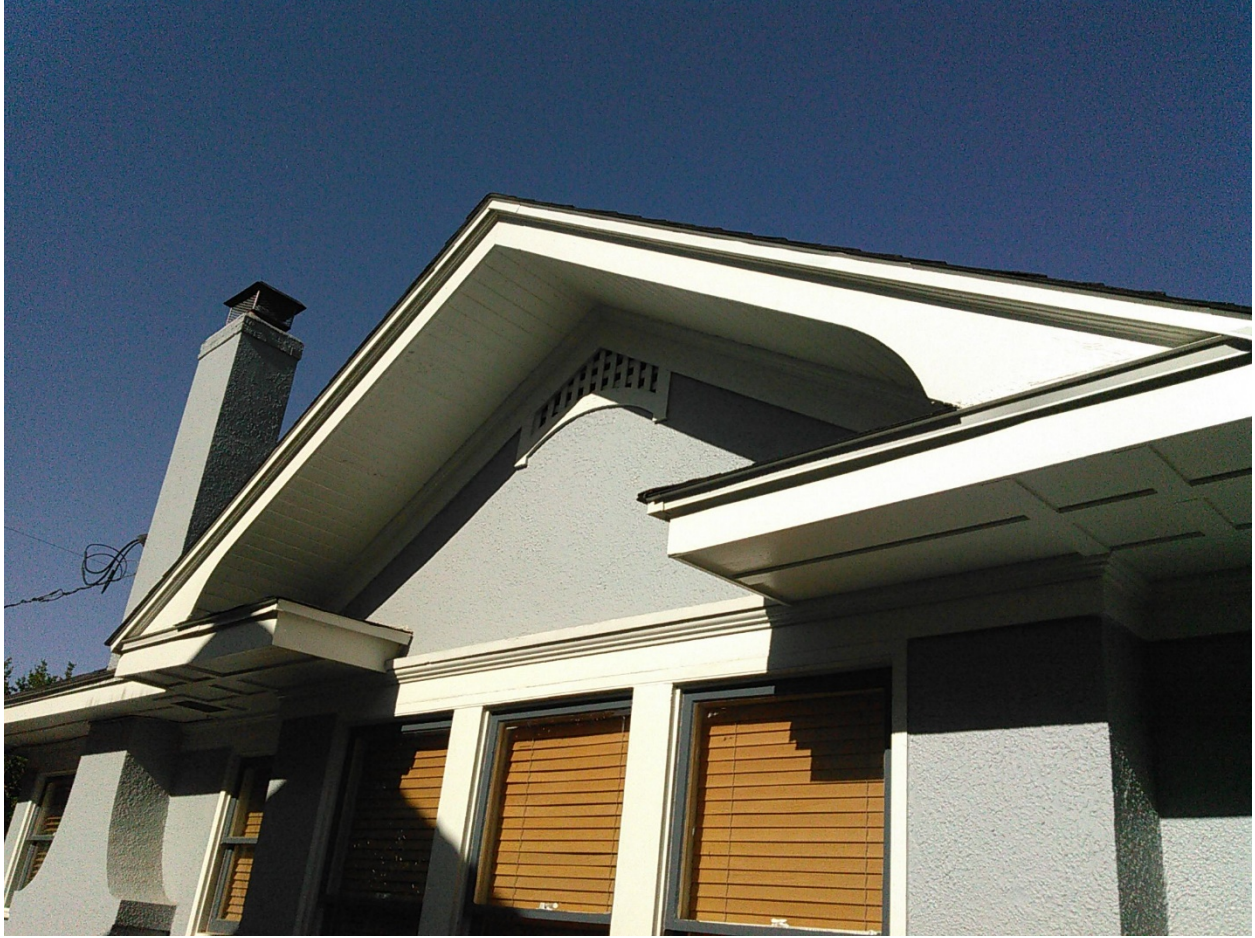
West side front gable with existing chimney in view.
