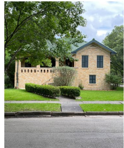
EXAMPLE OF AN ELEVATED HOME IN THE AREA
