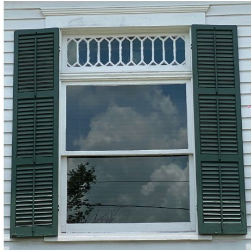
EXISTING DECORATIVE WINDOW TRIM
