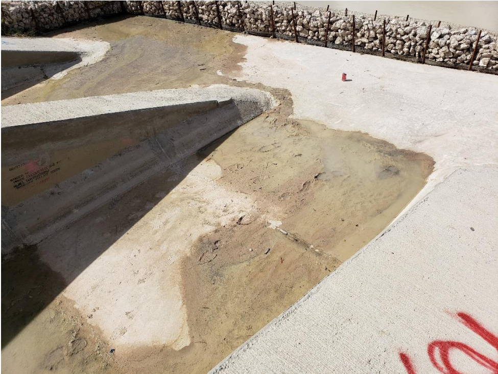
Remove Sediment from Outfall Structure
