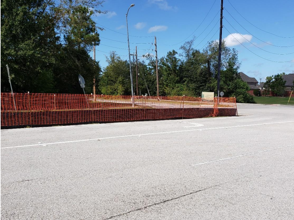
Median Protection on Woodland Hills Drive
