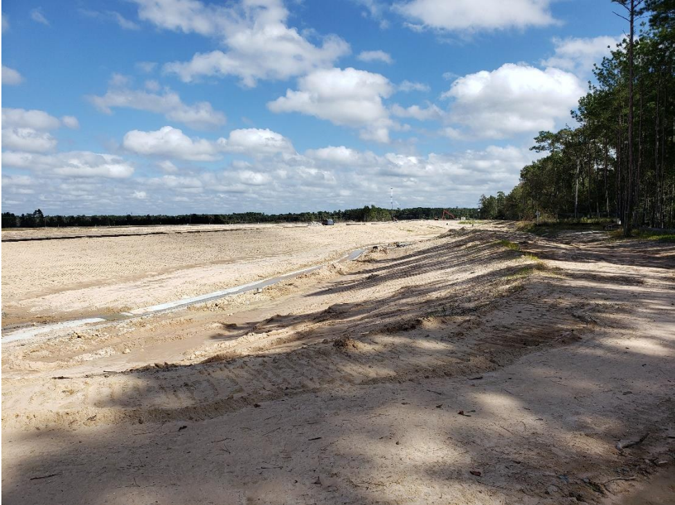
Detention Pond #2 Looking East
