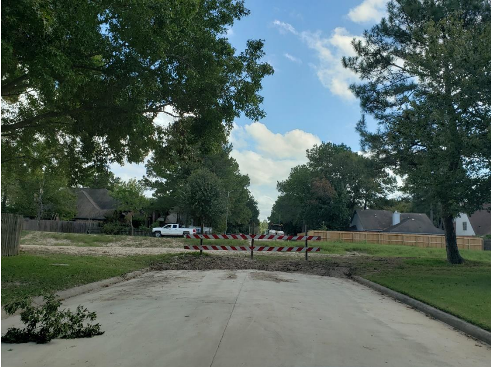
Remove Sediment and Stabilize Disturbed Area on Creek Manor Drive
