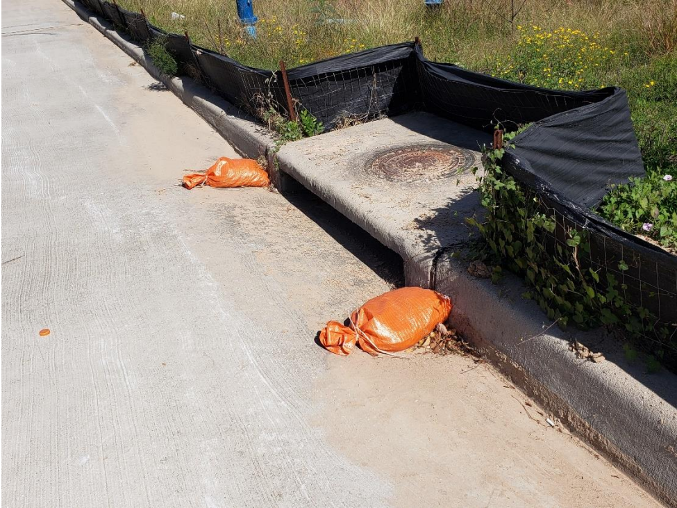
Inlet Protection Recently Maintained
