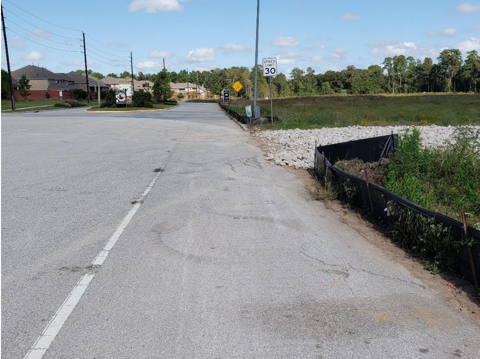
Construction Site Entrance on Woodland Hills Drive Note: Light tracking
