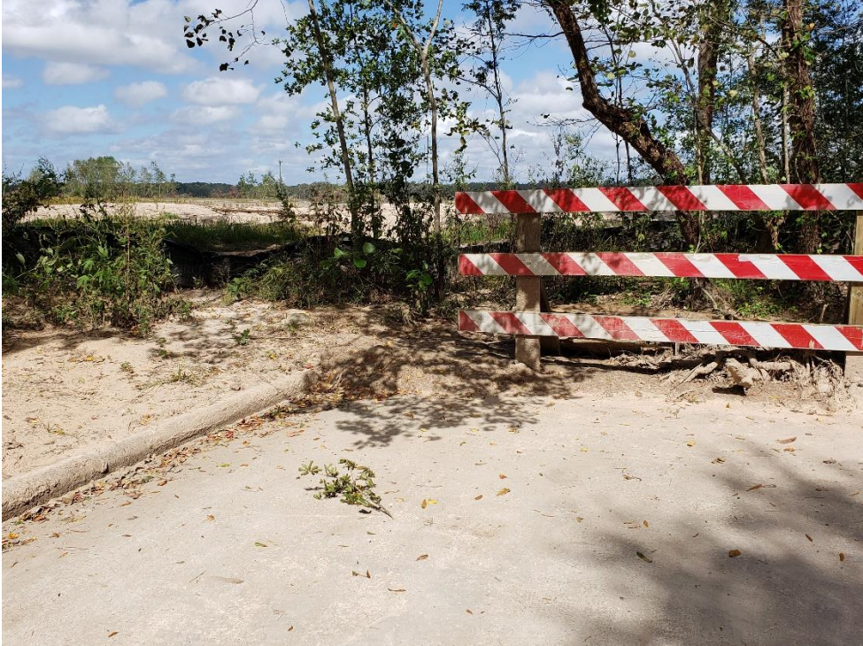
Remove Sediment, Stabilize Disturbed Area & Remove Debris on Village Springs Drive
