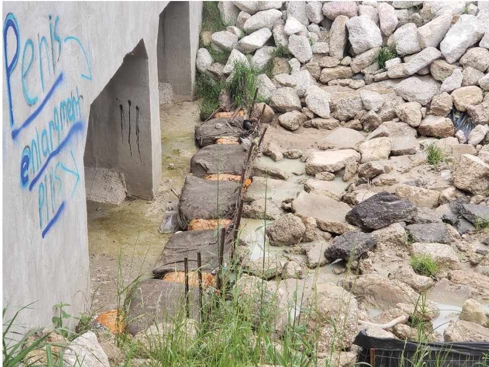
View of Outfall of Detention Pond #1 to Taylor Gulley Note: Hay Bales are well maintained
