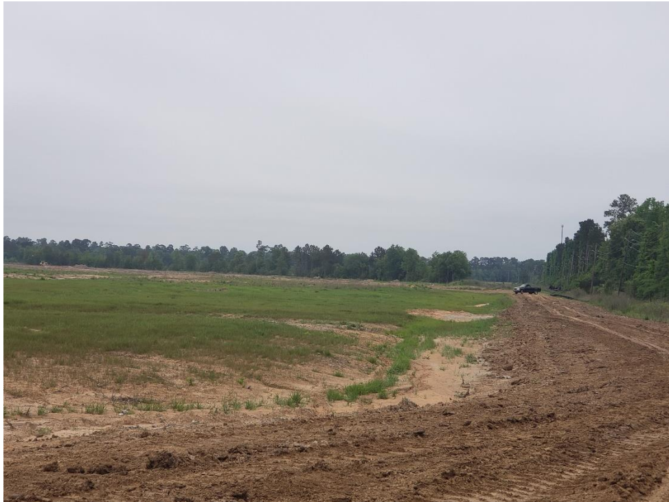
View of Northern Clear-cut Area Looking East Note: Area has been hydro-mulched and is partially stabilized
