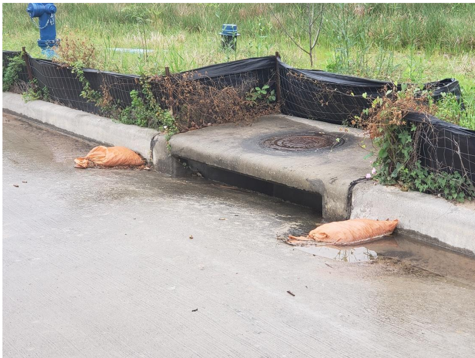
Inlet Protection on Woodland Hills Drive
