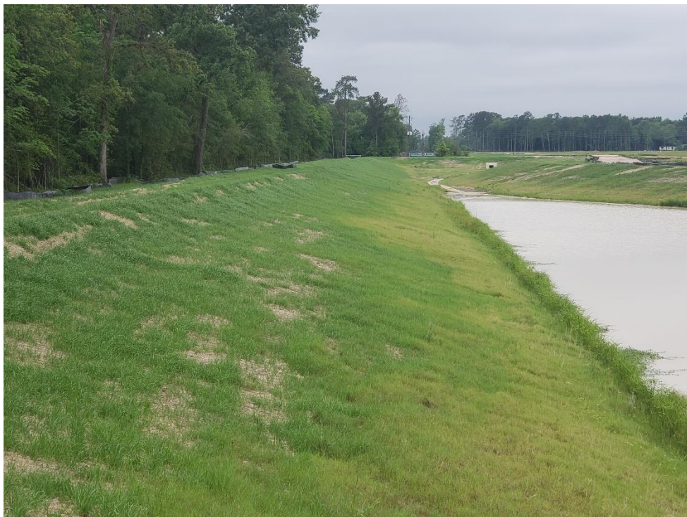
Berm between Detention Pond #1 and #2
