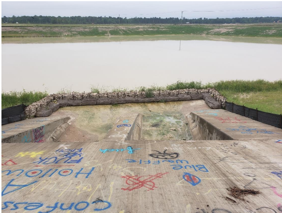
View of Upstream Outfall Structure from Detention Pond #1 to Taylor Gulley Note: Hay bales are in place and well maintained
