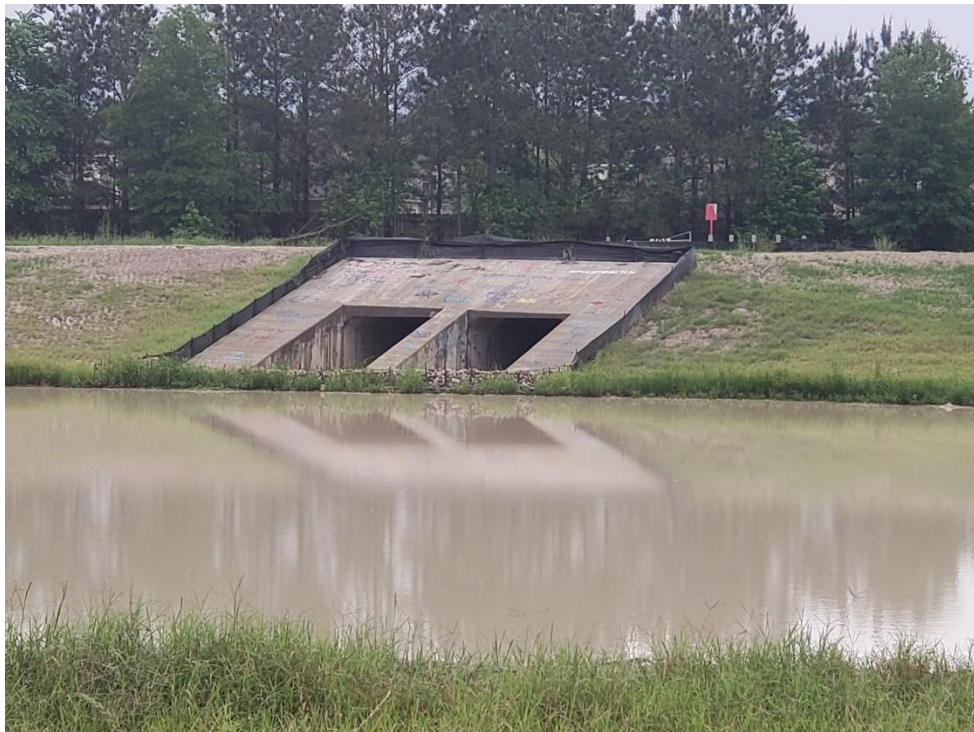
View of Upstream Outfall Structure from Detention Pond #1 to Taylor Gulley
