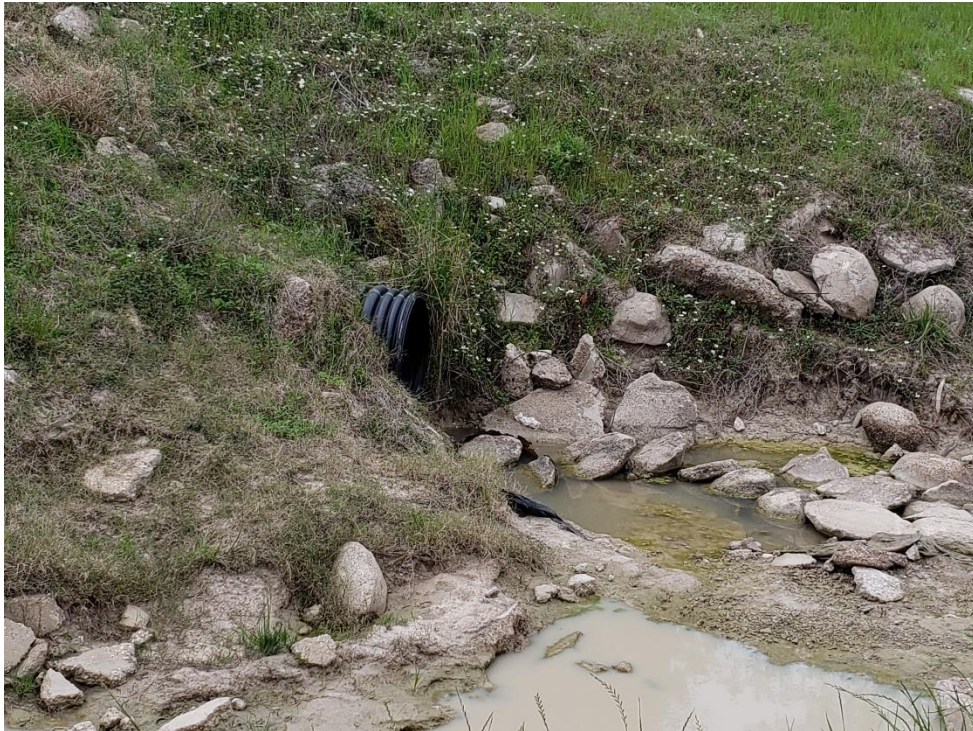
View of Montgomery County Flood Control Ditch Outfall to Taylor Gulley Note: No Discharge
