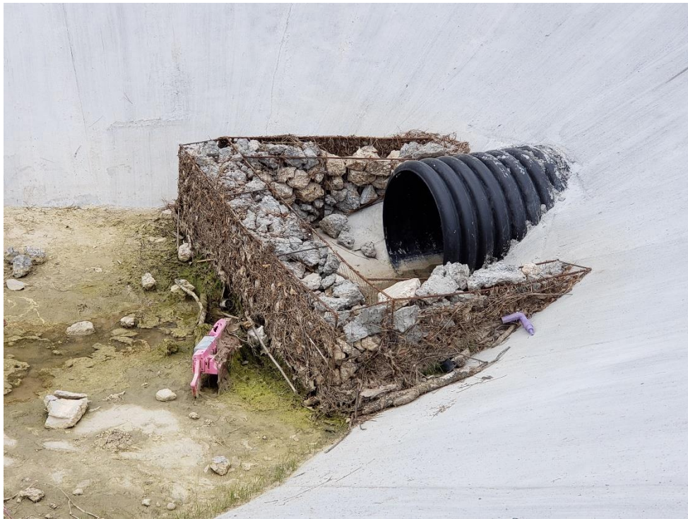
View of Montgomery County Flood Control Ditch Outfall to Taylor Gulley
