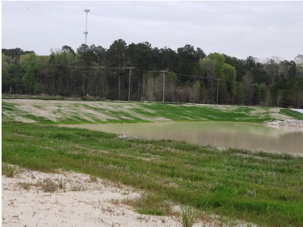
Detention Pond #1 Side Slopes are Dressed and Stabilized with Hydro-Mulch Note: Bare areas require attention
