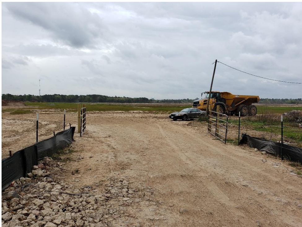
View of New Gate at Construction Entrance on Webb Road
