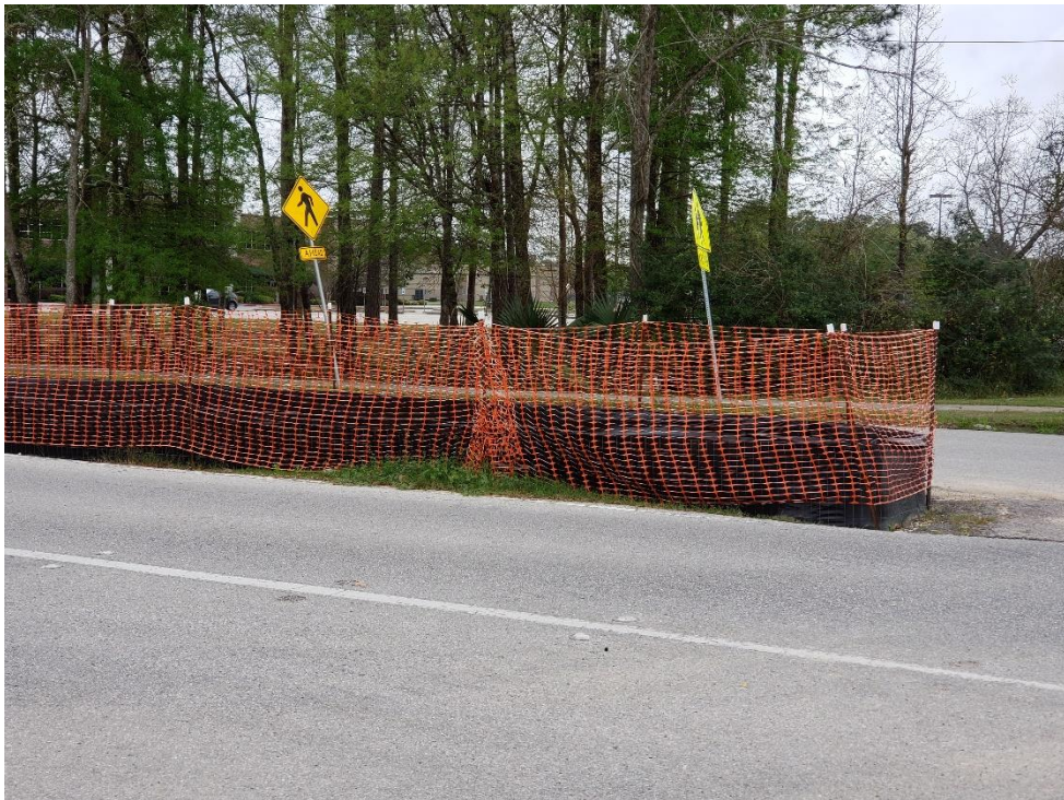
Median Protection on Woodland Hills Drive
