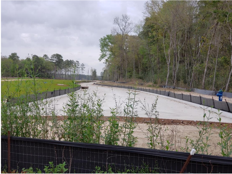
New Street to be Connected to Woodland Hills Drive
