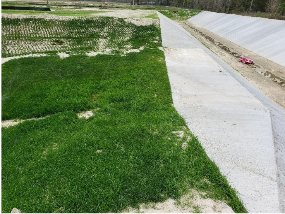
View of Overflow from Montgomery County Flood Control Ditch to Detention Pond #1 Note: This area has been re-stabilized with Hydro-Mulch
