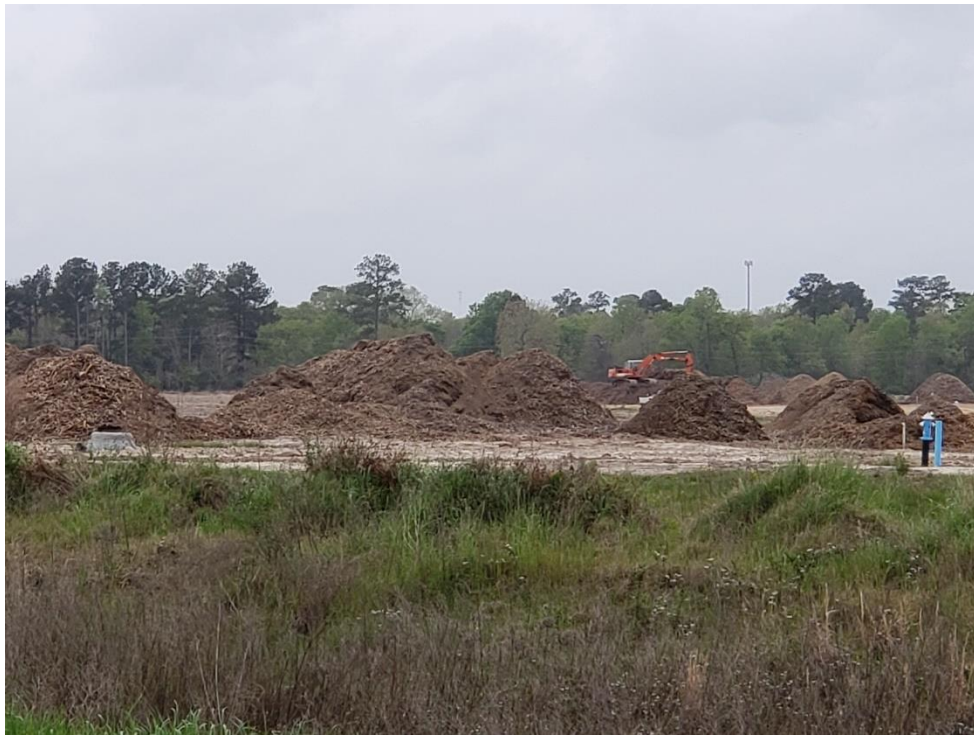
Mulch Gathered for Transport and Disposal Off Site
