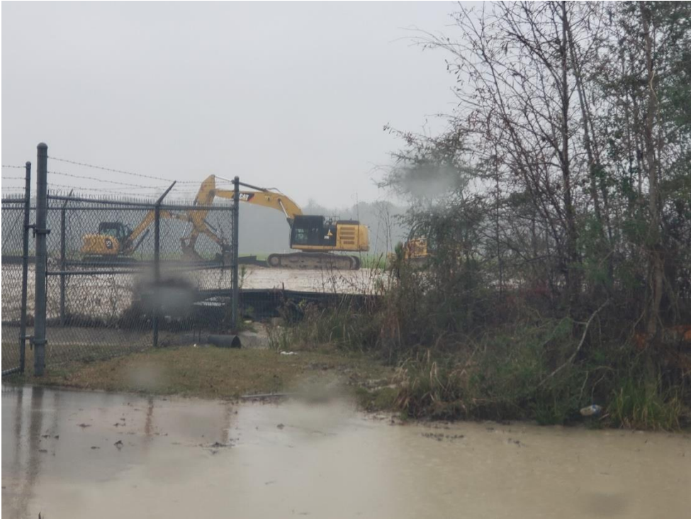
View of Former Equipment Staging Area
