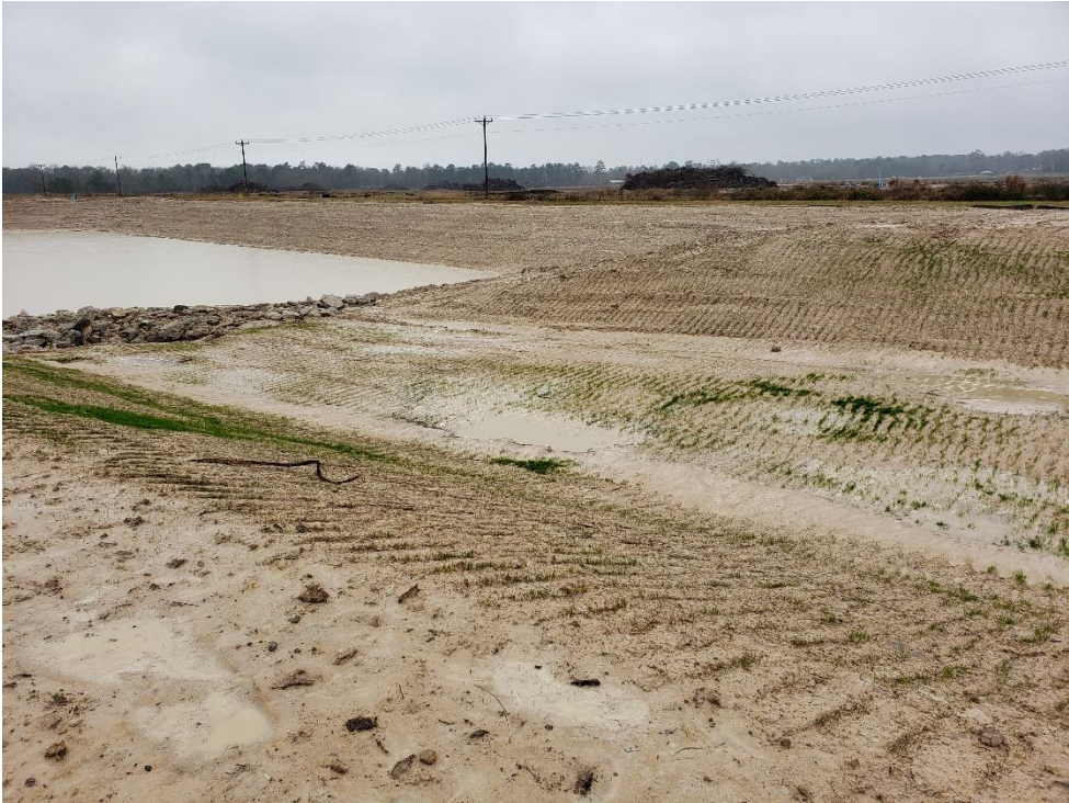
View of Overflow from Montgomery County Flood Control Ditch to Detention Pond #1 Note: Grass seeds are germinating
