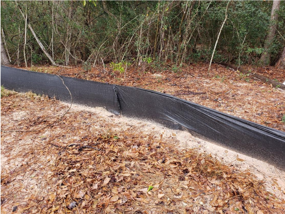
View of Silt Fencing in Good Condition
