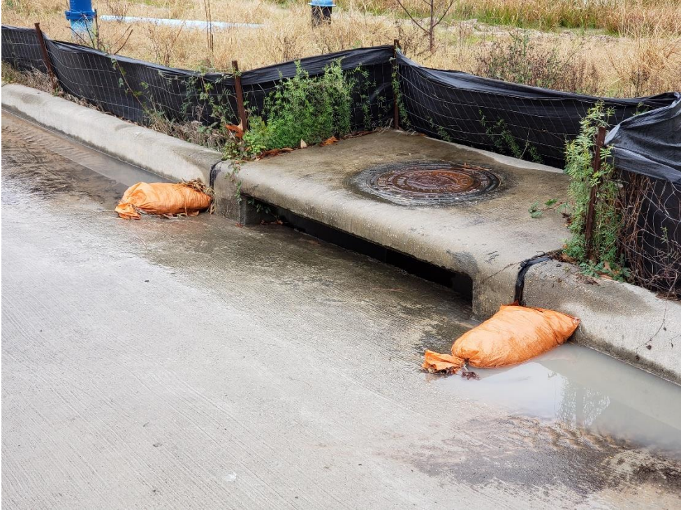
Inlet Protection on Woodland Hills Drive
