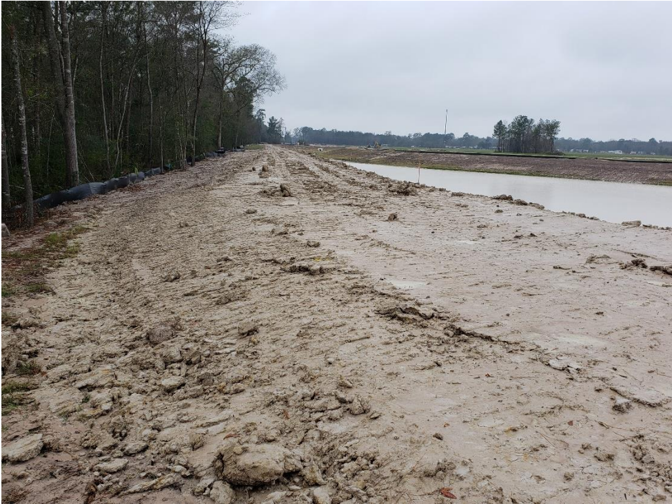
View of New Berm at Detention Pond #1 Looking West
