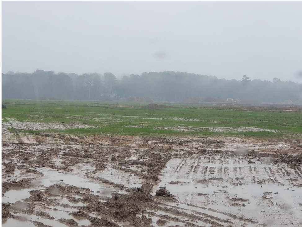
View of Northern Clear-cut Area Looking Southeast Note: All trees and brush have not been chipped
