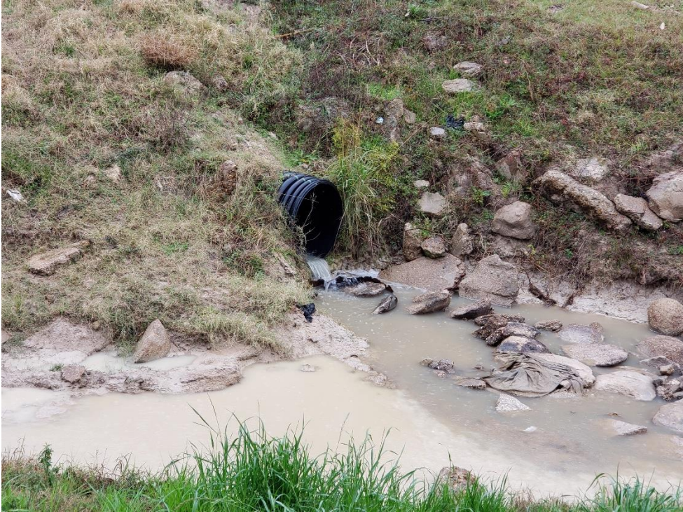
View of Montgomery Flood Control Ditch Outfall to Taylor Gulley
