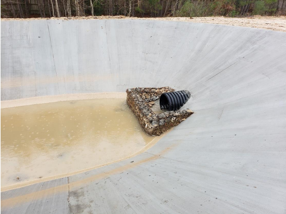
Upstream Outfall of Montgomery County Flood Control Ditch to Taylor Gulley
