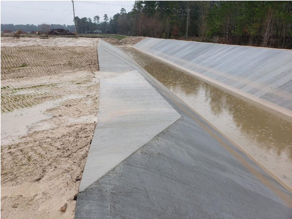
View of Montgomery County Flood Control Ditch with Concrete Slopes
