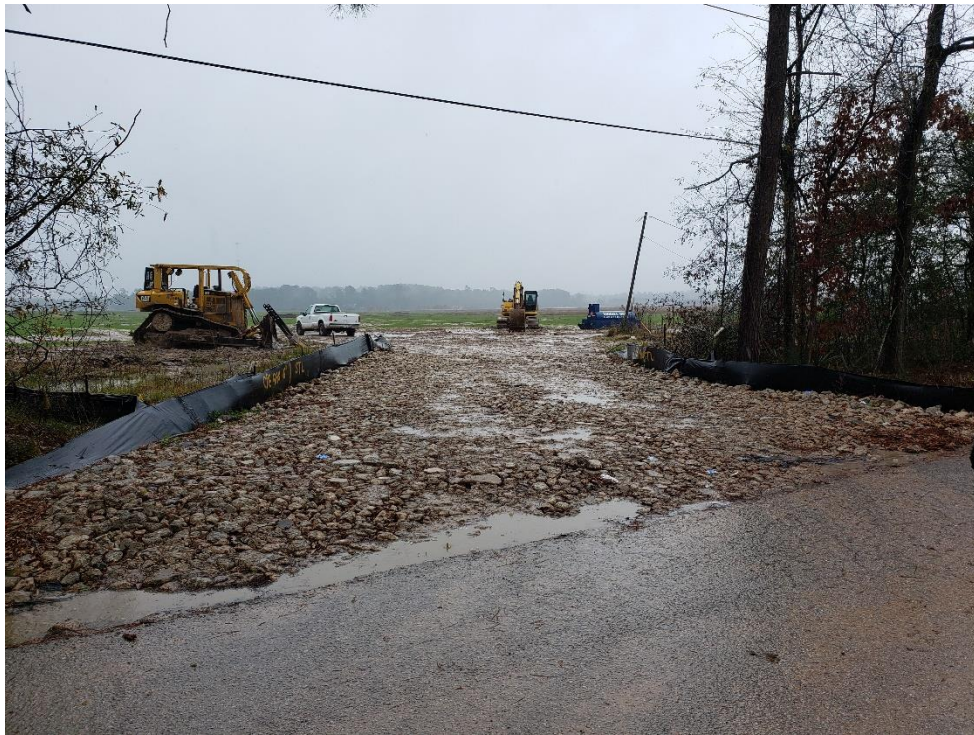
View of Construction Entrance on Webb Road Note: Light tracking
