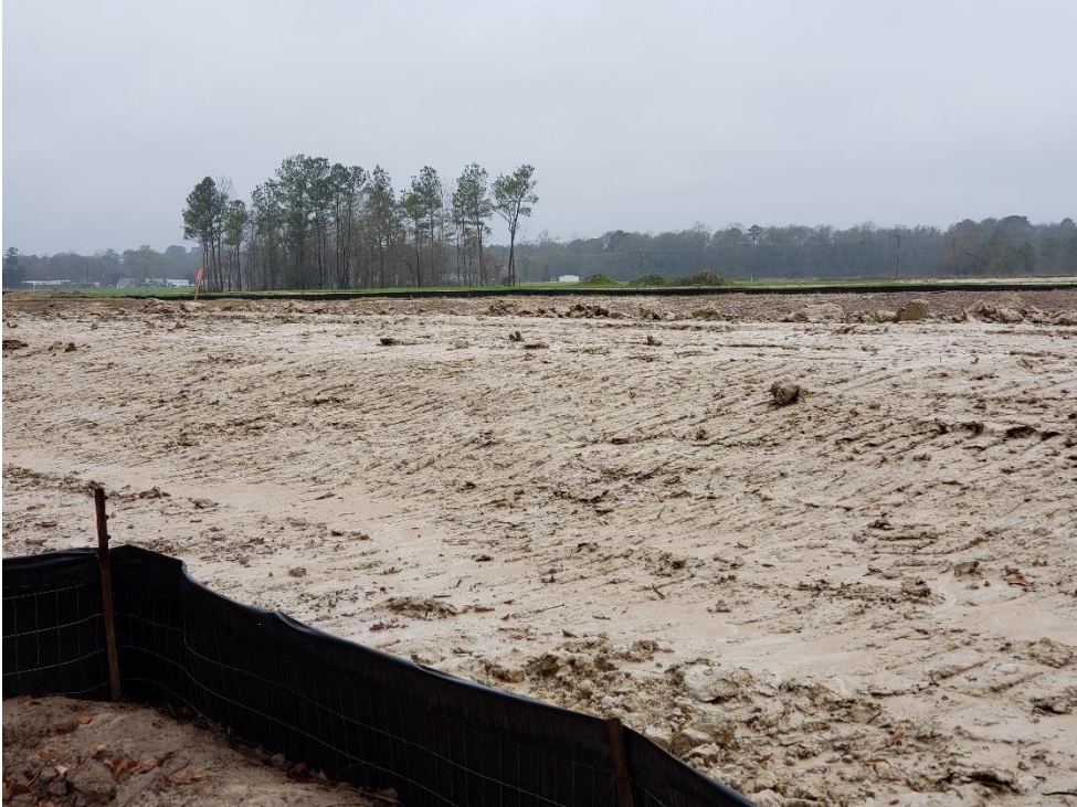
View of New Berm Between Detention Pond #1 and #2
