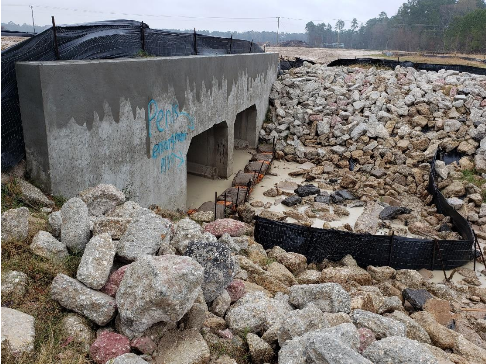
View of Outfall of Detention Pond #1 to Taylor Gulley Note: Hay Bales are well maintained
