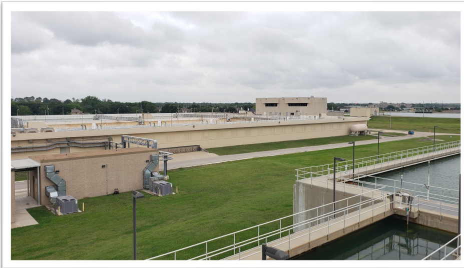
Southeast Water Purification Plant
